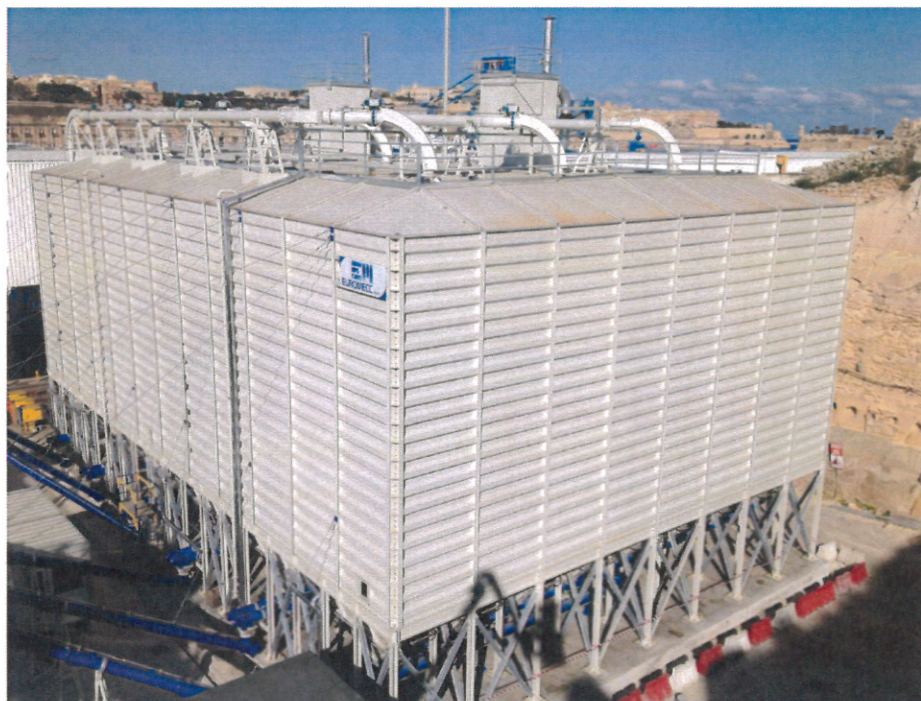
Photo 5 – Actual Installation, Silo Facilities
