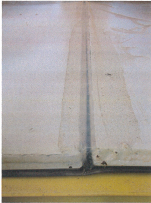
Photo 7: Sealer applied along internal seams to protect self adhesive foam placed in between steel panels along joints prior to tightening bolts
