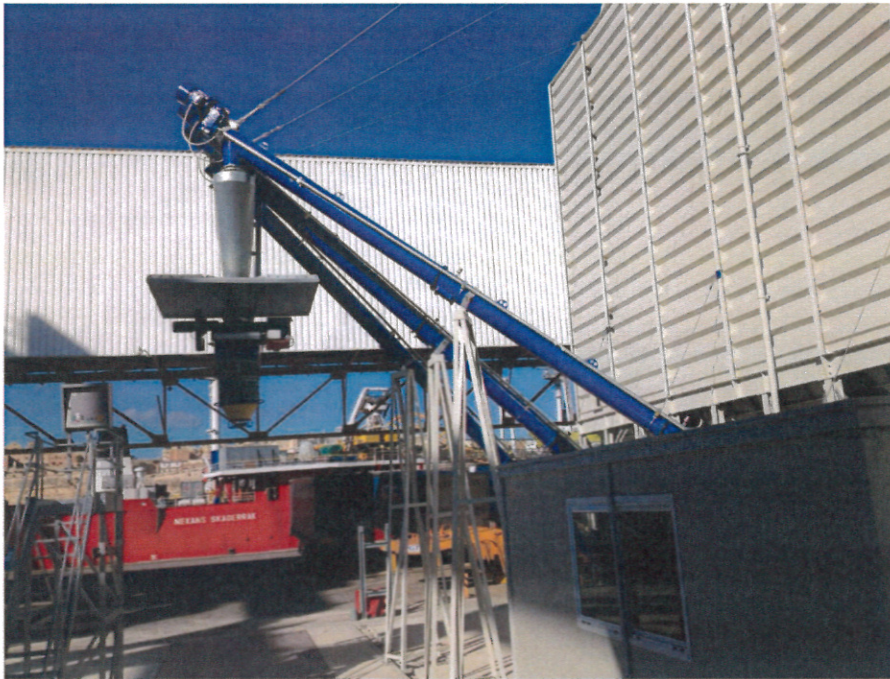
Photo 3 – Actual Installation, Inclined Screw Conveyors and Telescopic Unloading Bellows
