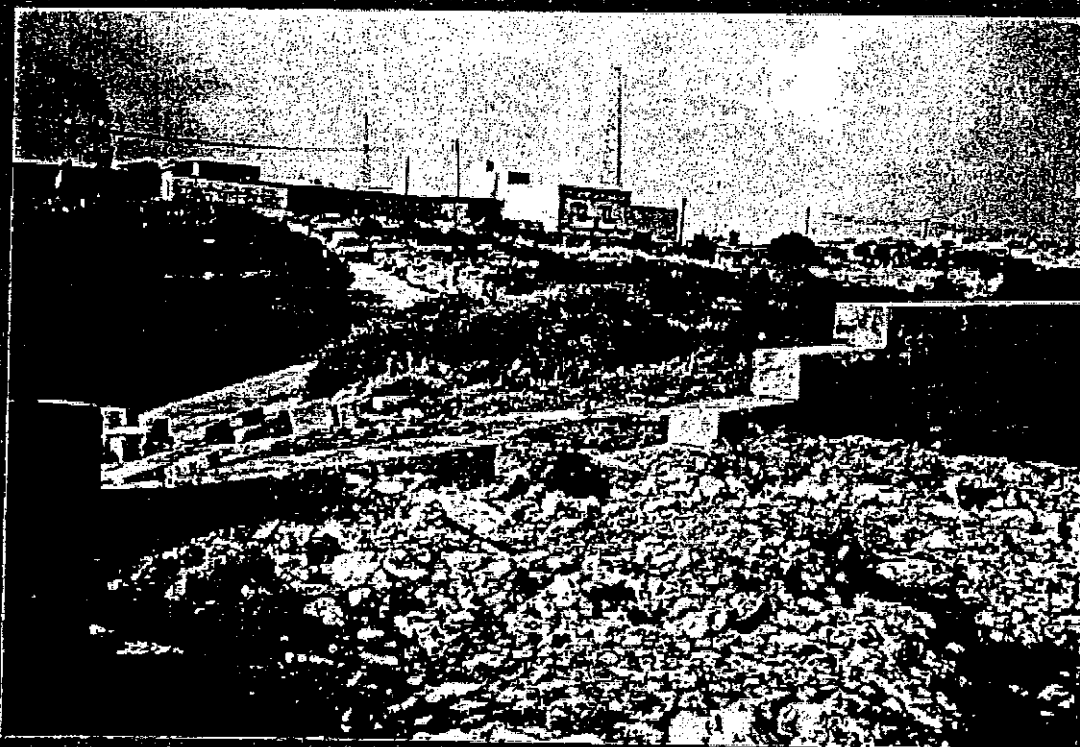
Fig. 3. Missing part of parapet wall along land-front fortifications.
