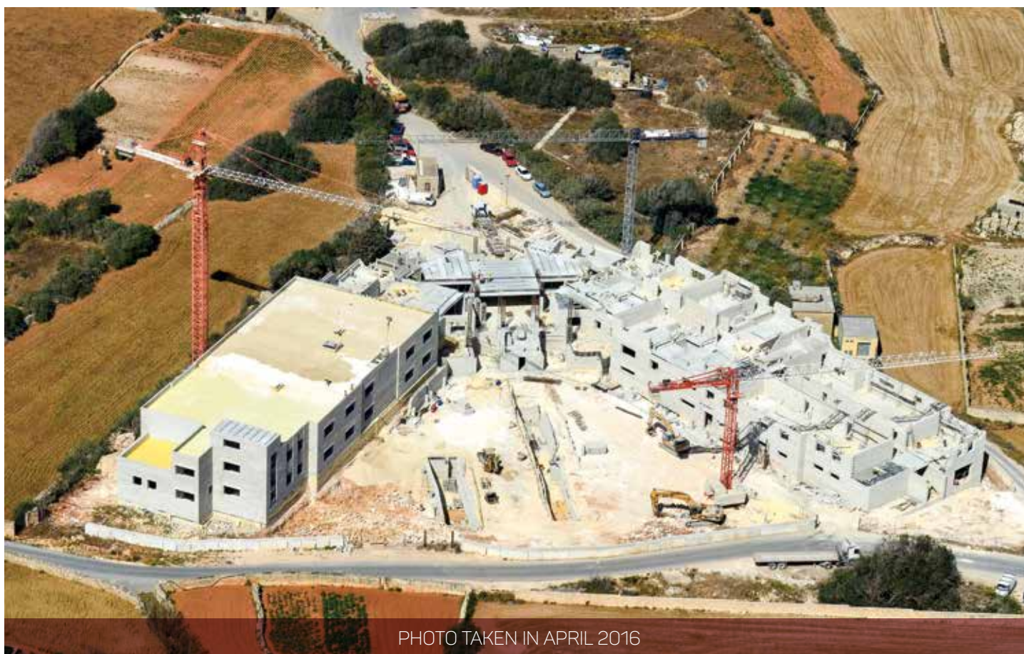
PHOTO TAKEN EARLY IN CONSTRUCTION
