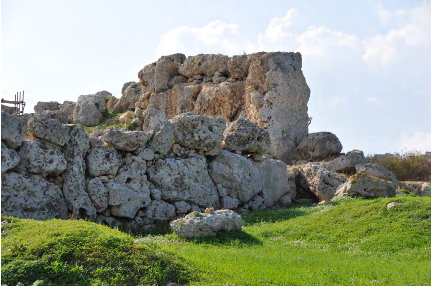
40. North-east external wall - detail
