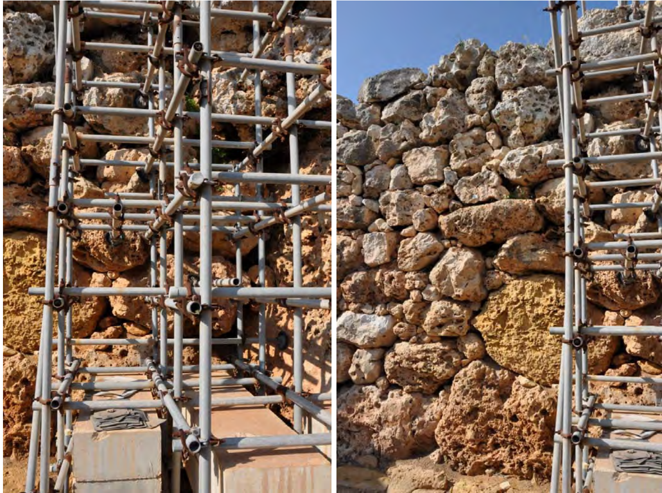
32 , 33. Detail of scaffolding – junction between apse 6 and 7 – discontinuity in masonry assembly
