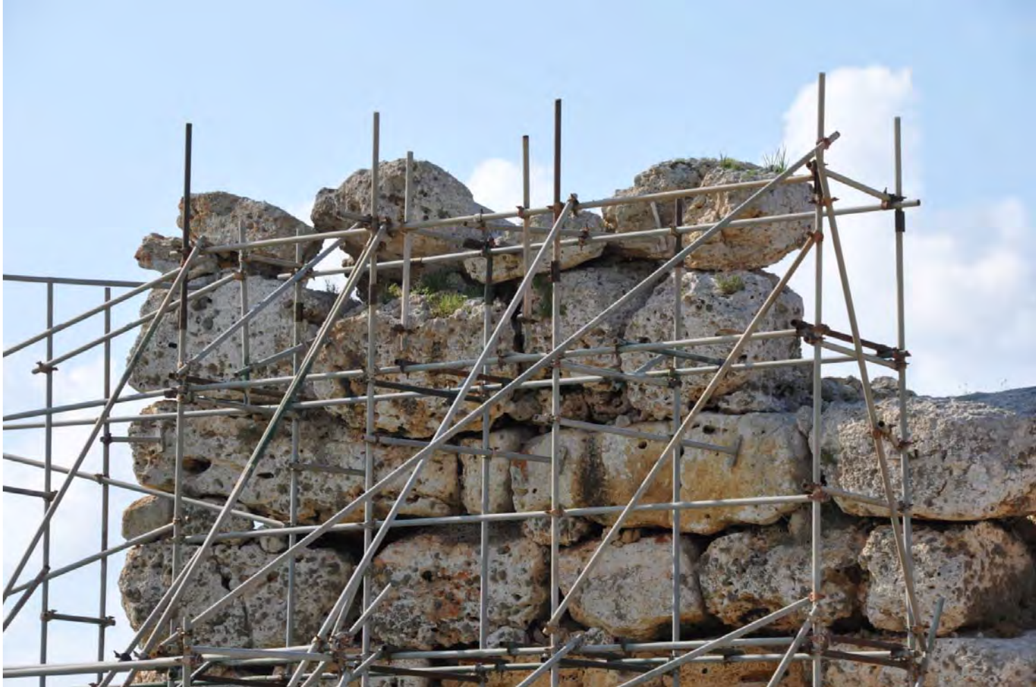
15. Propped south-east facade – close-up
