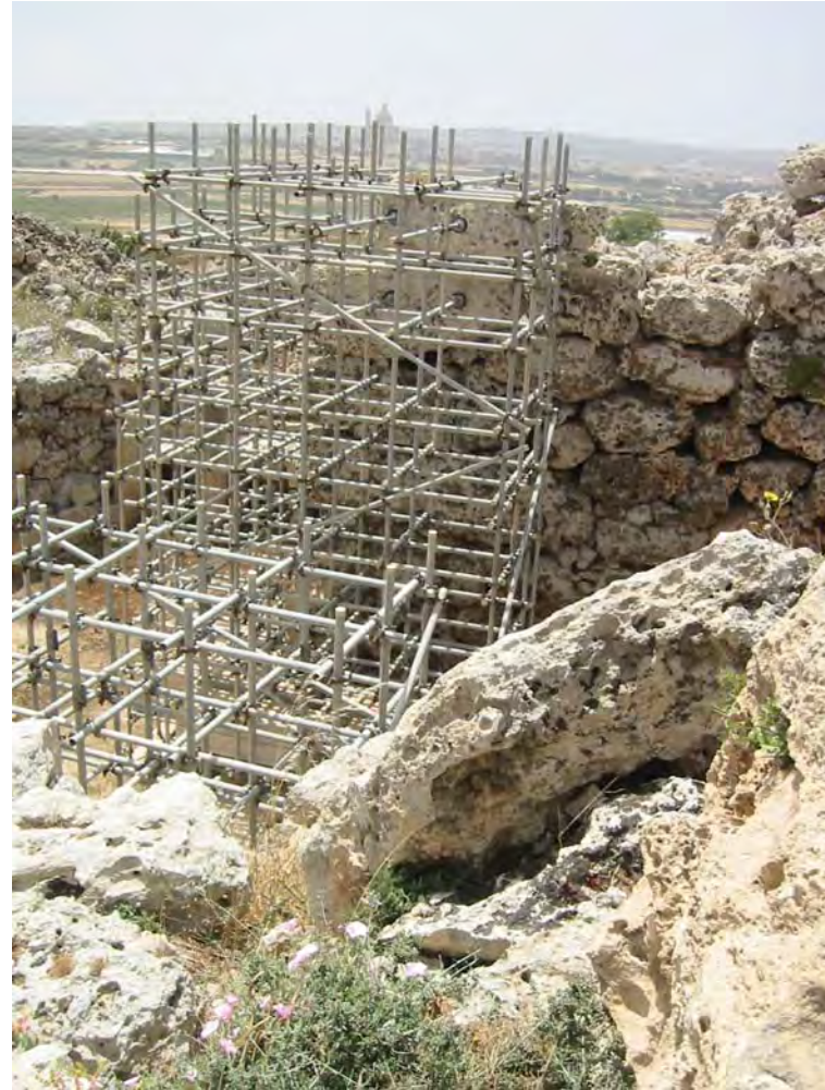
77. 2005 view of South Temple – propping at Apse 7
