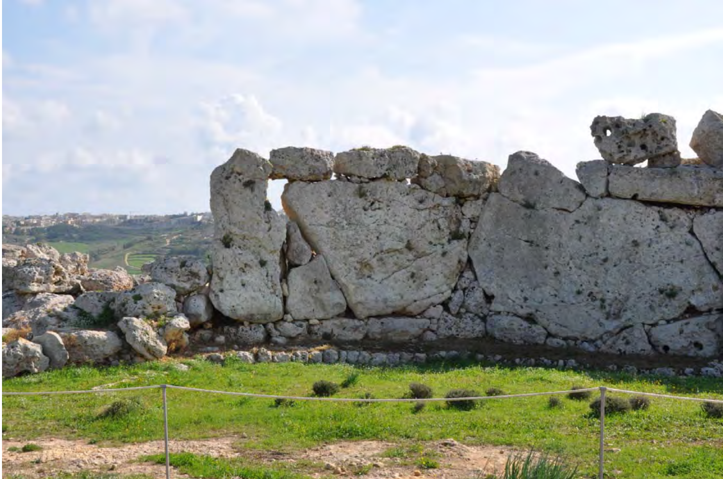
5. North-west external wall - detail
