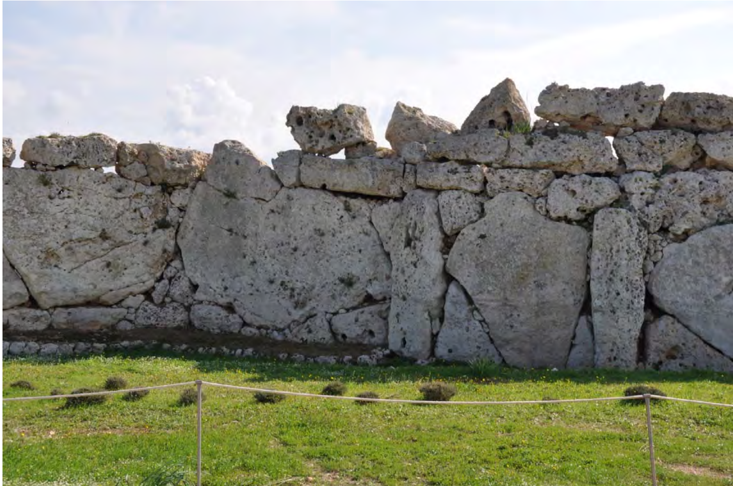
6. North-west external wall - detail
