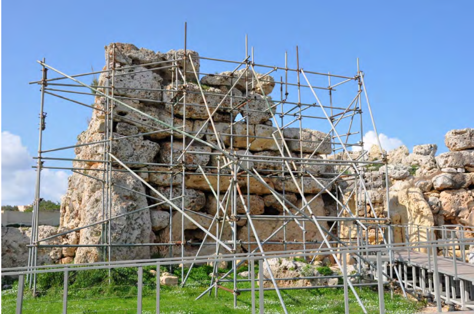
13. Propped south-east facade – detail
