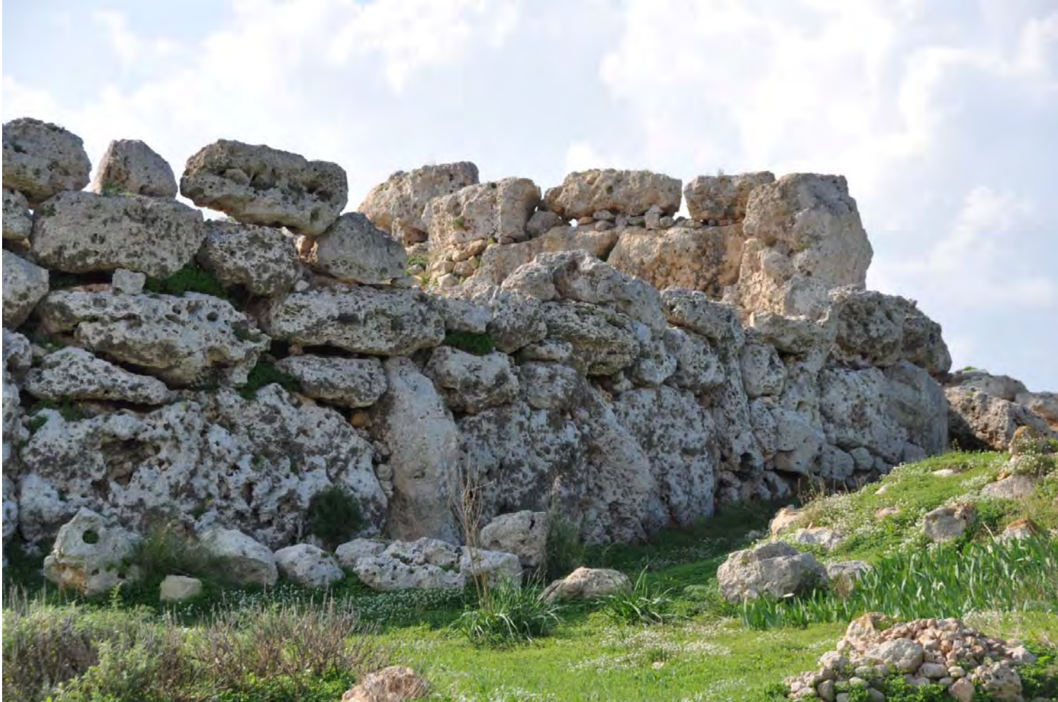
39. North-east external wall - detail
