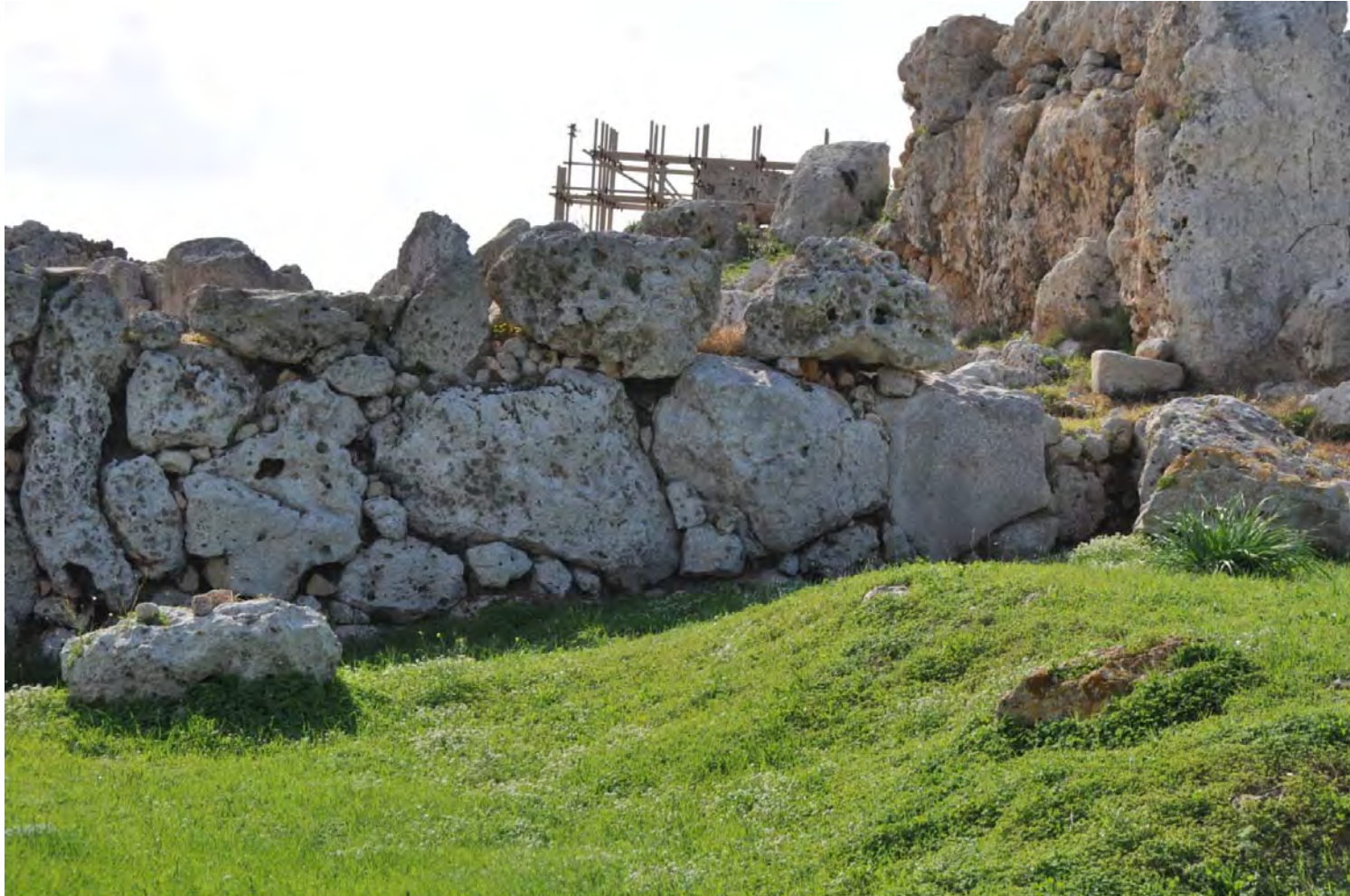
41. North-east external wall - detail
