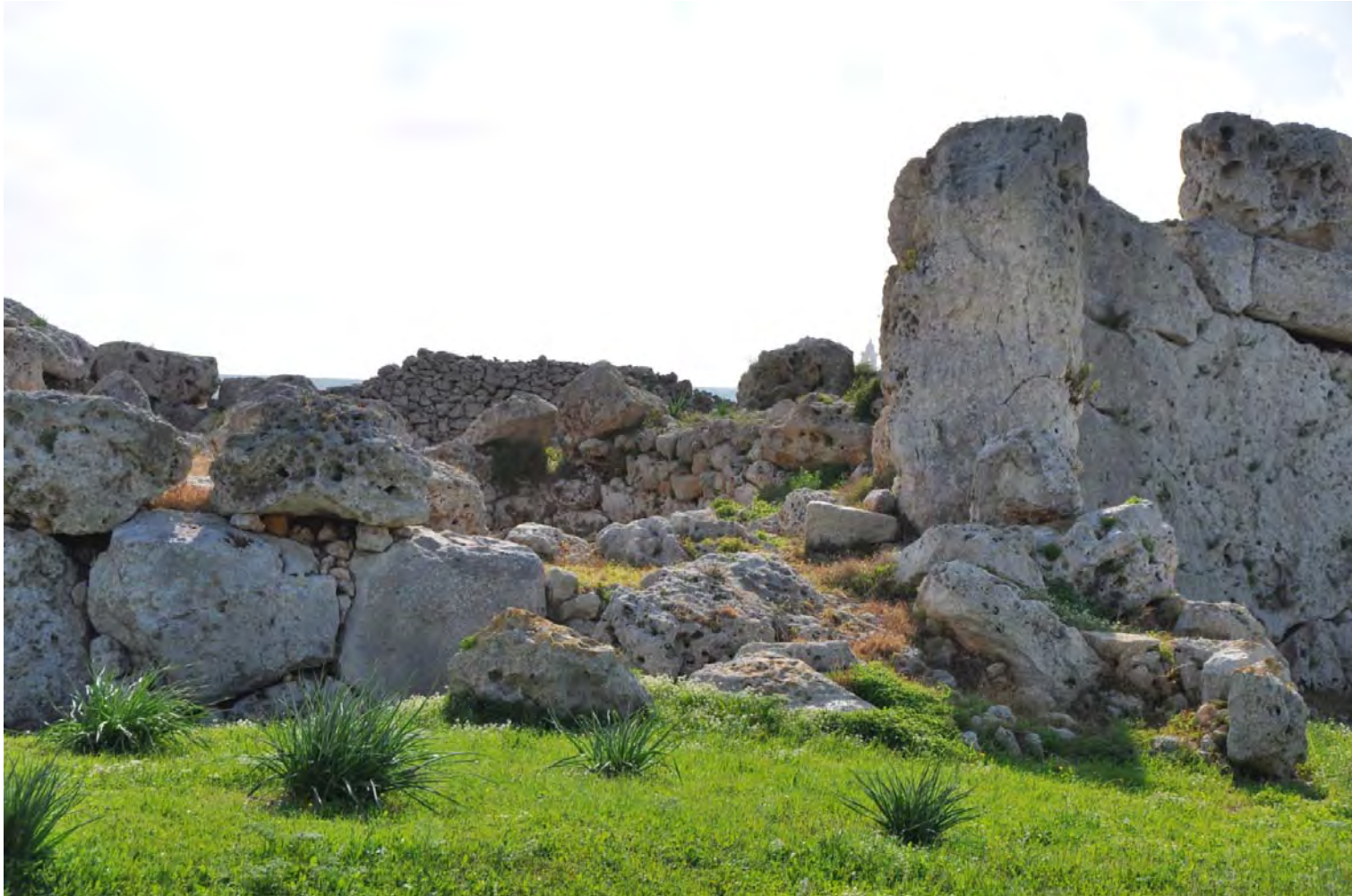
42. North-east external wall - detail
