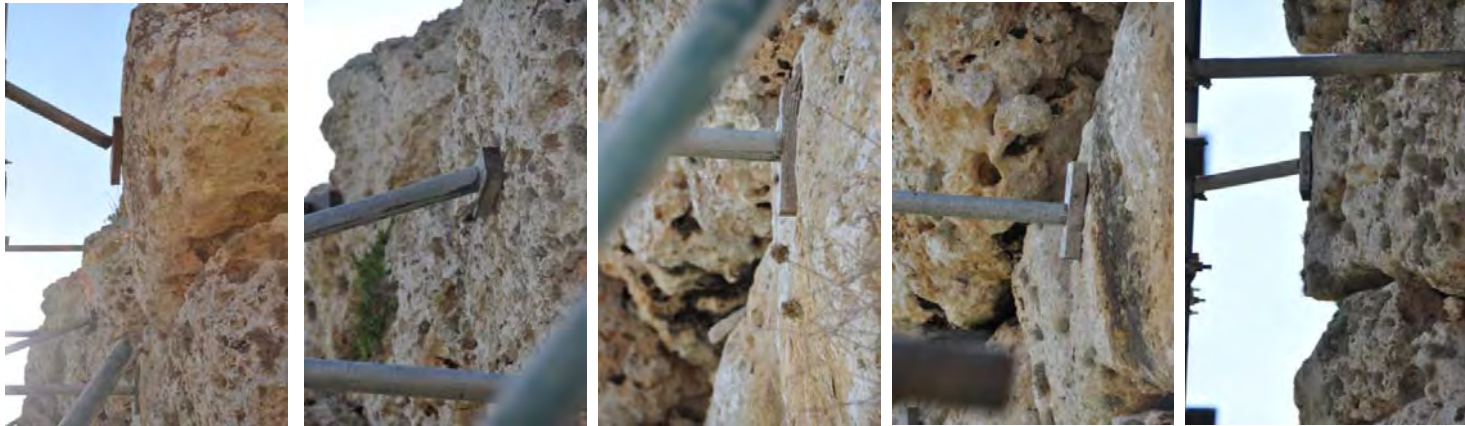
19. Propped south-east facade – close-up of contact between scaffolding and stones
