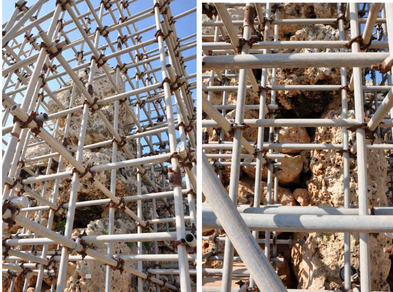
28 , 29. Detail of scaffolding – junction between apse 6 and 7 – discontinuity in masonry assembly
