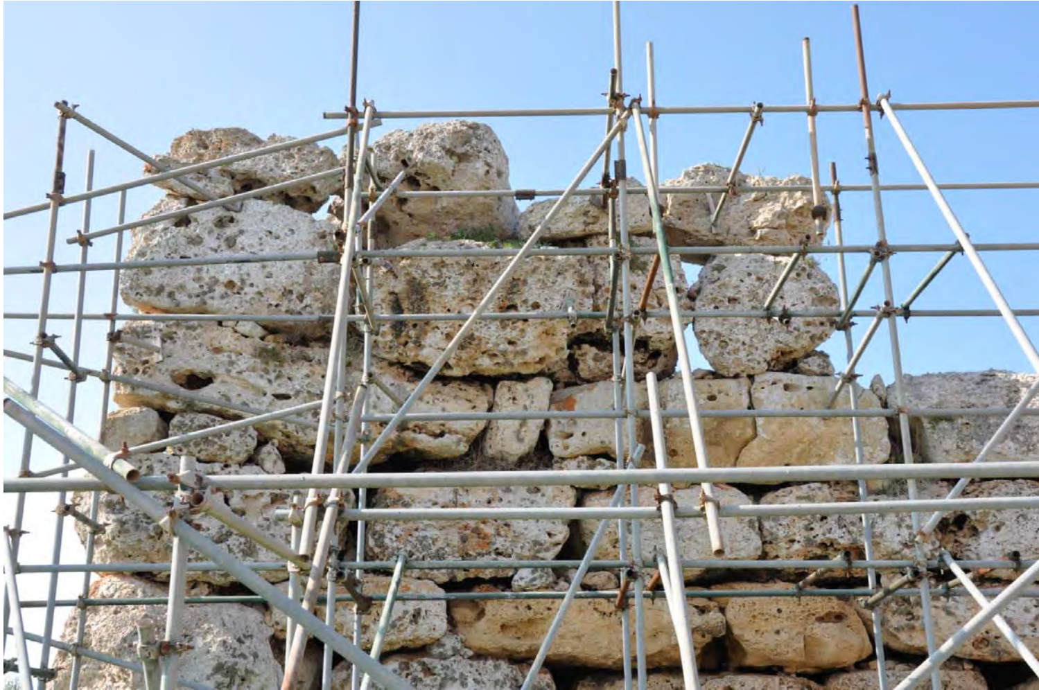
16. Propped south-east facade – close-up
