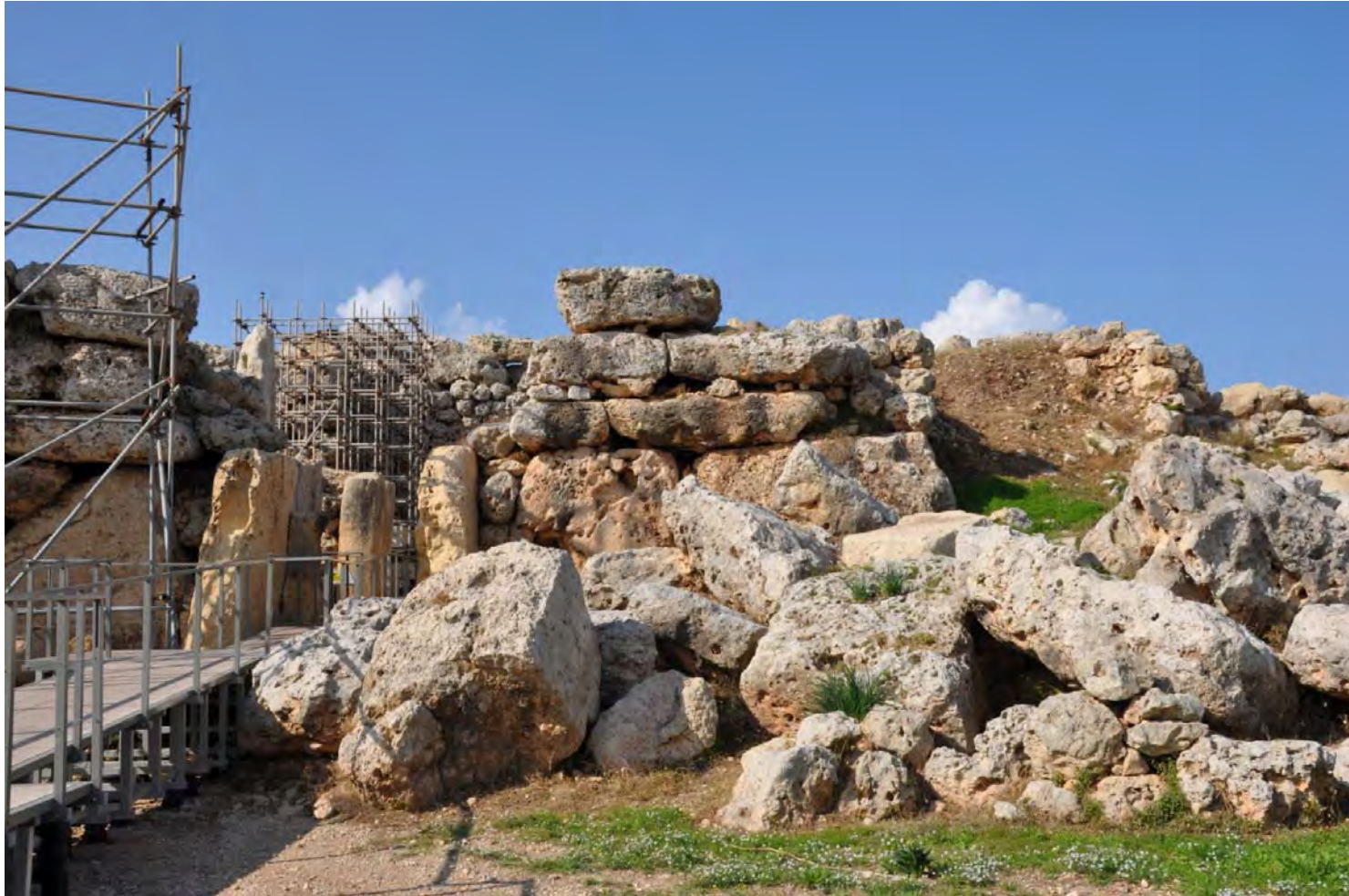
14. Previous collapse between temples – south-east facade detail
