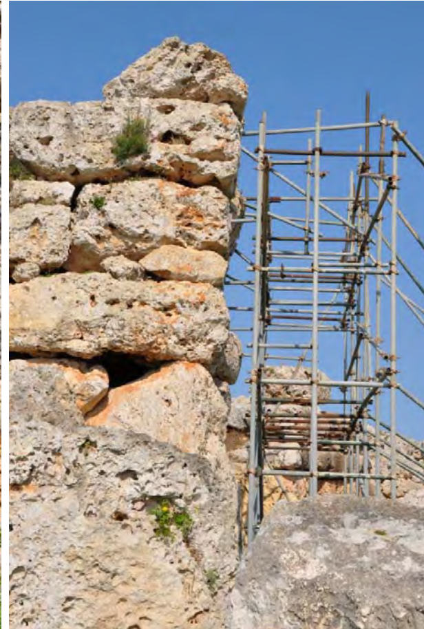
9. Props against south-west facade – detail
