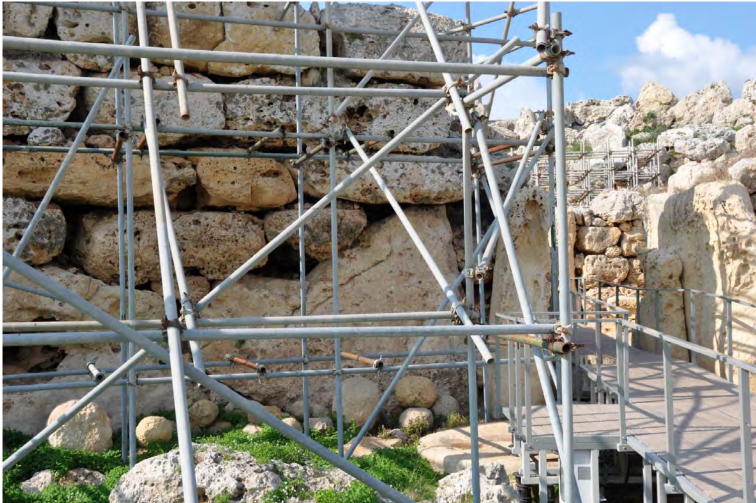
18. Propped south-east facade – close-up
