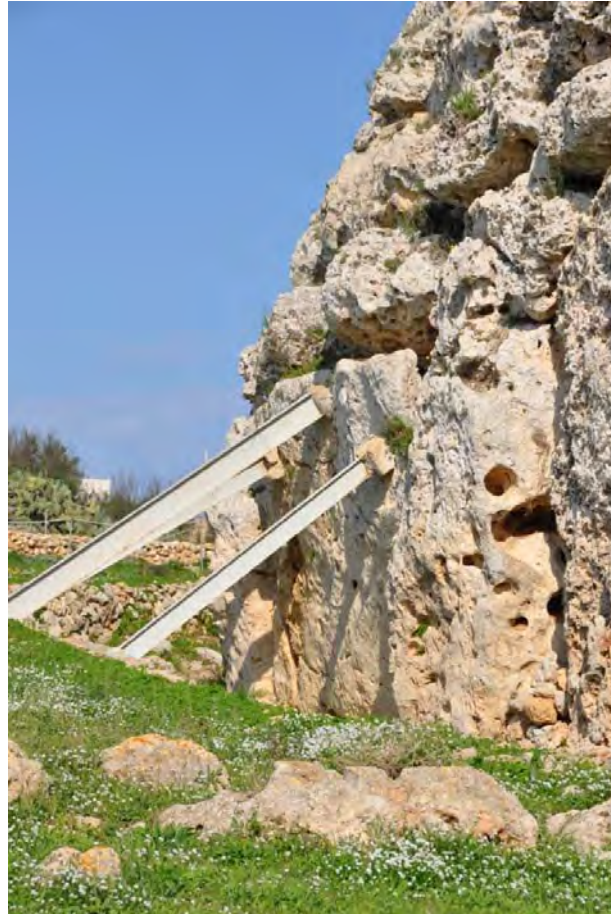
8. Props against west external wall – detail
