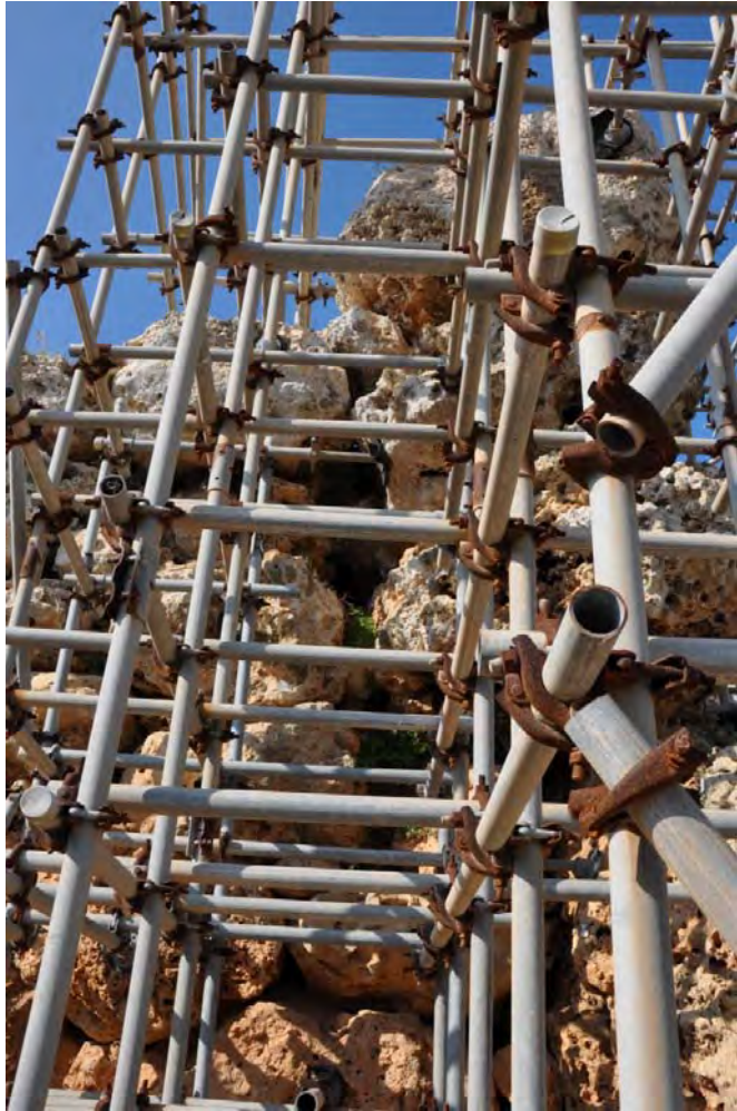
30 , 31. Detail of scaffolding – junction between apse 6 and 7 – discontinuity in masonry assembly
