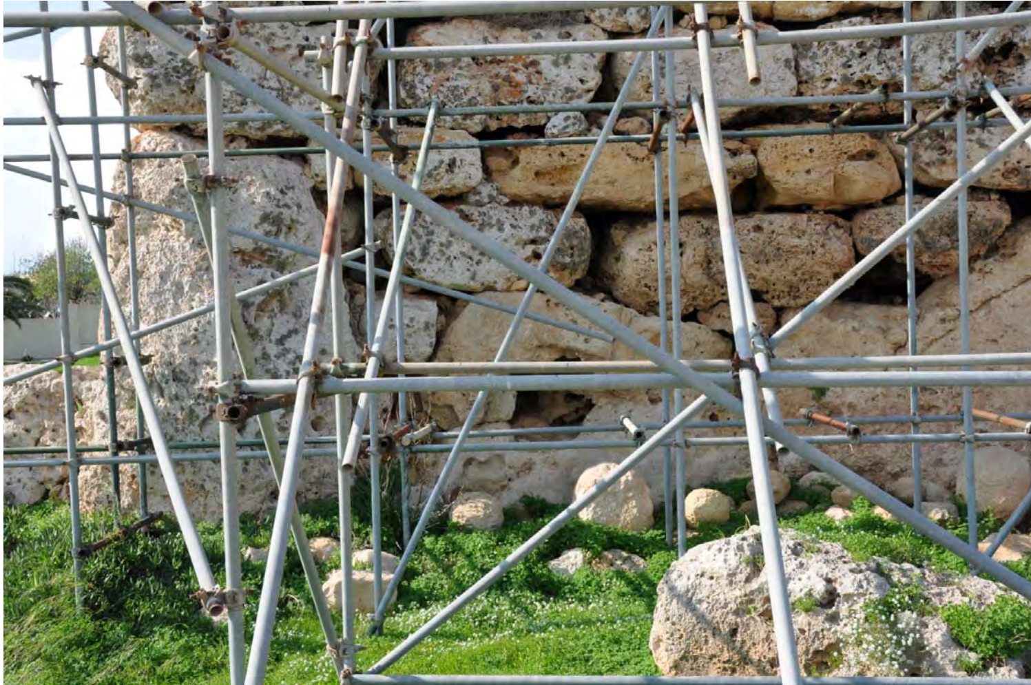
17. Propped south-east facade – close-up
