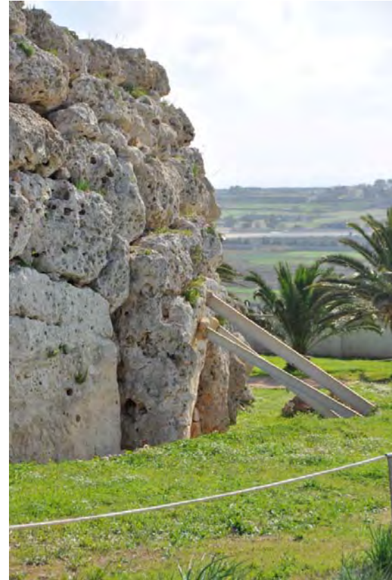
44. Propped external wall – detail
