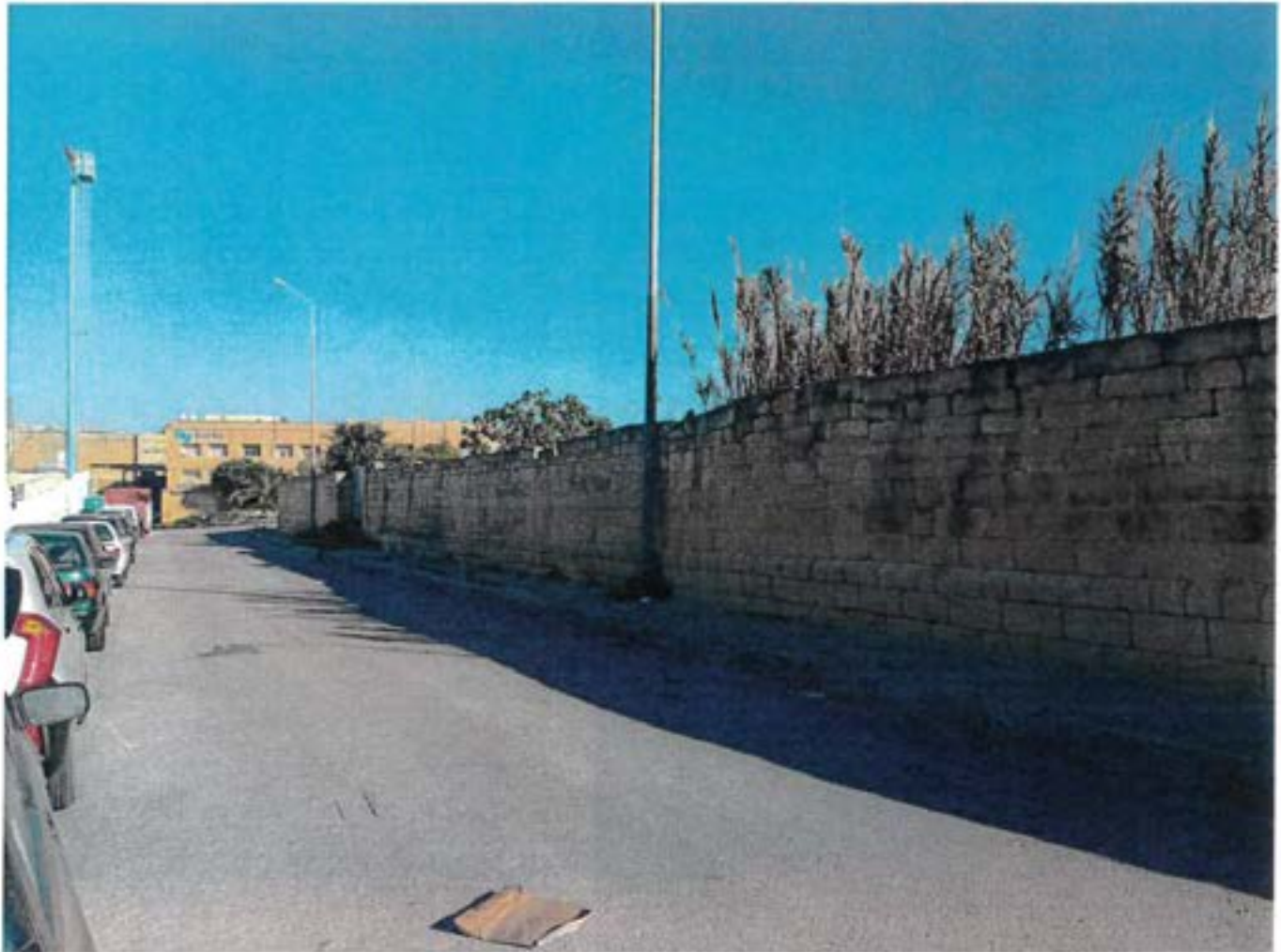
Photo 1: Photo showing the stretch of road together with the boundary wall, all making part of the land in question.
