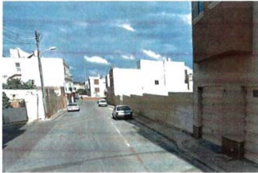
Photo 1: View of the site along Triq Salvu Sacco
