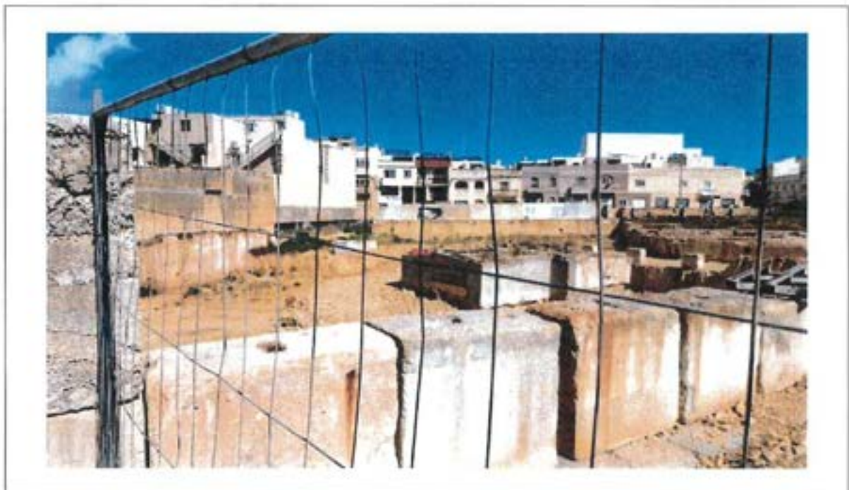
Photo 2: excavation works in progress, however no updated PA application apparently ongoing!
