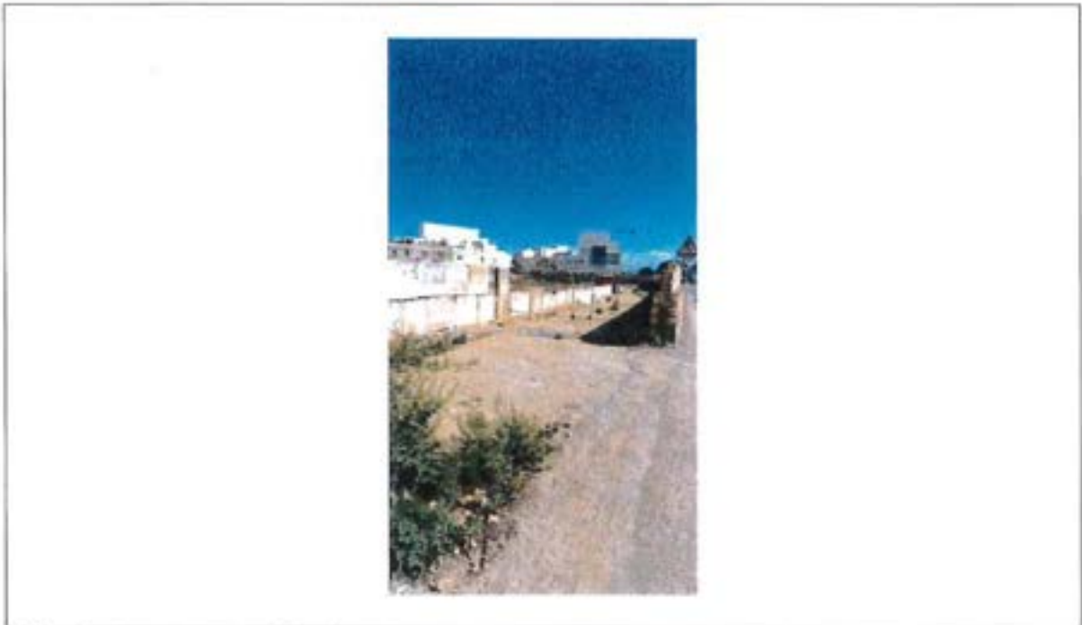
Photo 1: access to construction site.
