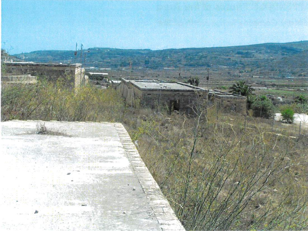
Image 3: Barracks built at different levels along slope
