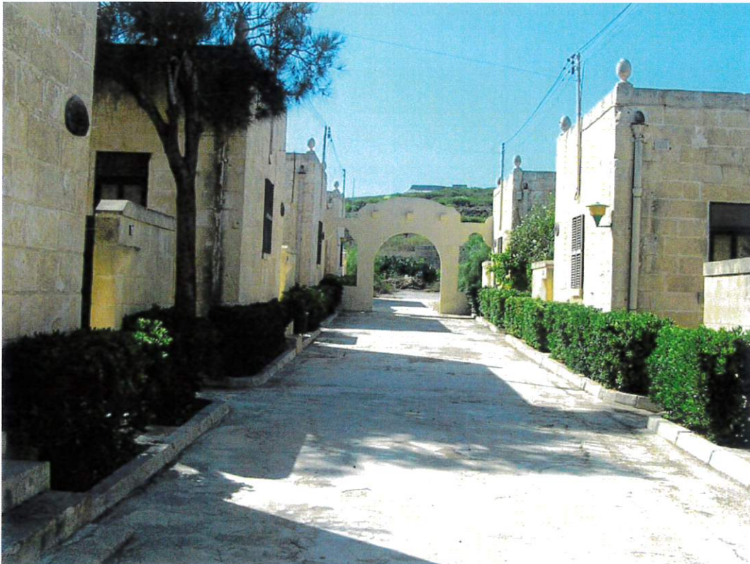
Image 16: Former Barrack Blocks (C24)
