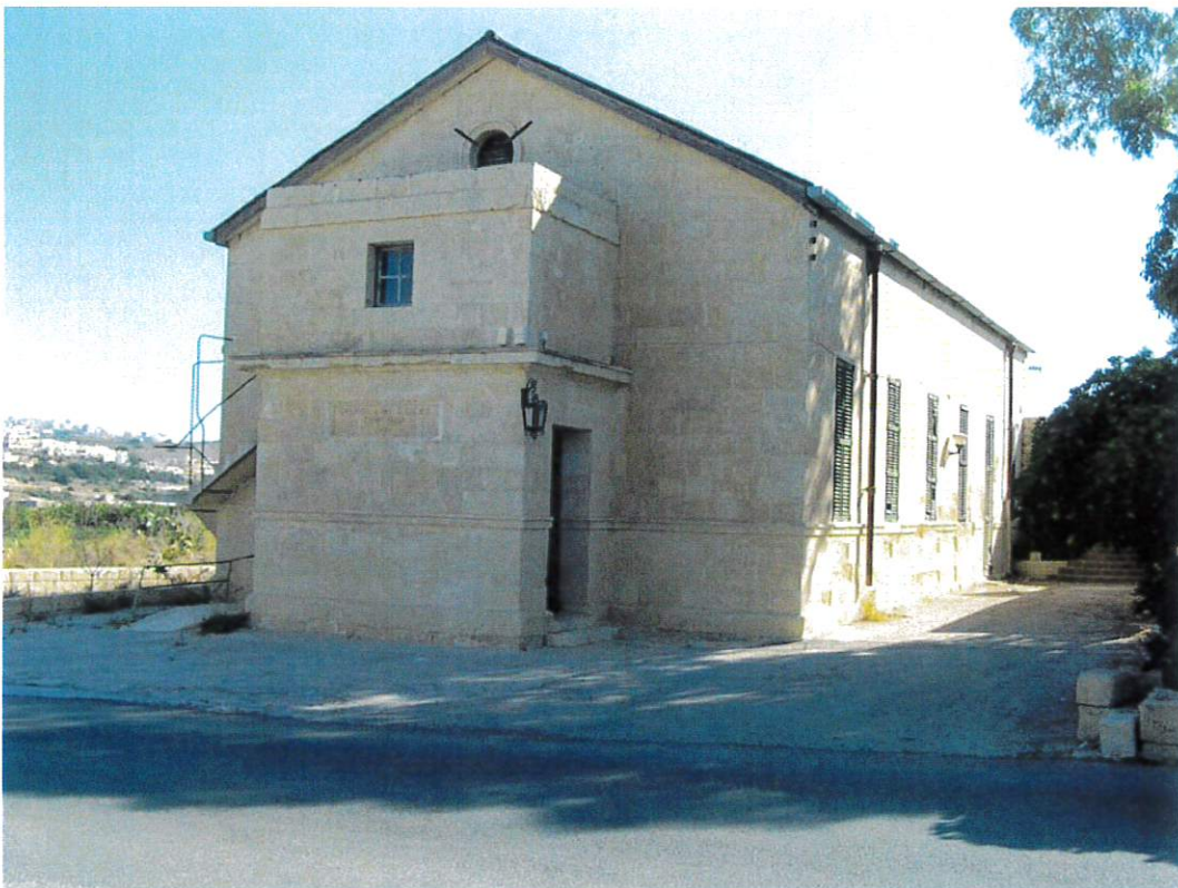
Image 10: Former Church/ Cinema built in 1916 (C20a)
