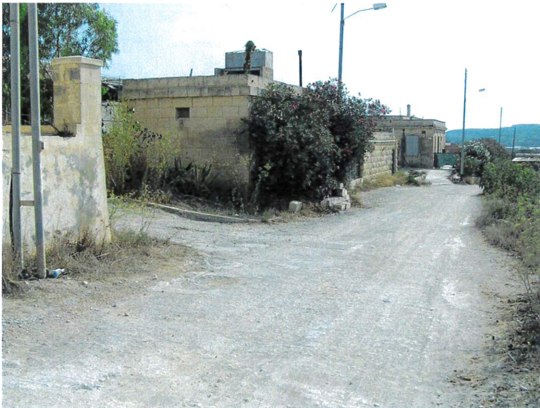
Image 4: View towards former Washhouse/ Stores
