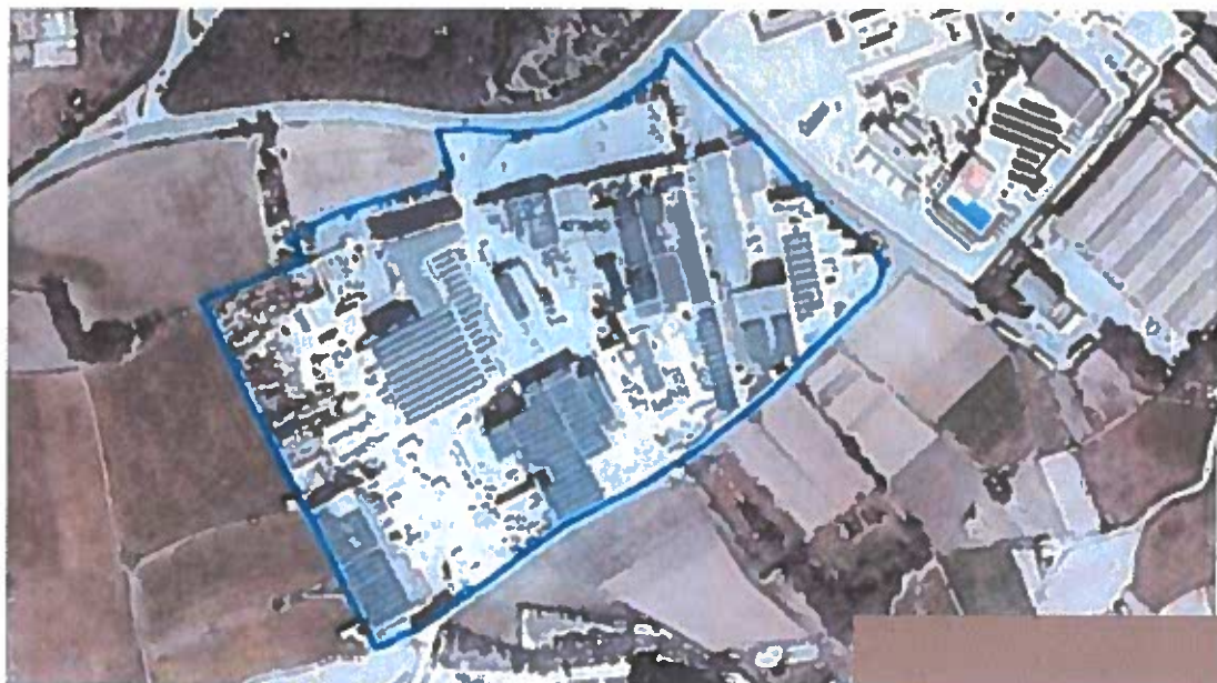
Figure 1 Aerial photograph with superimposed site boundary
