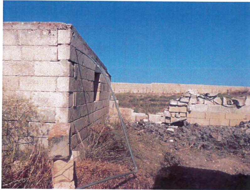
Photo 15: South elevation of structure No 13, as indicated in table 1, and its outside area next to structure No 19
