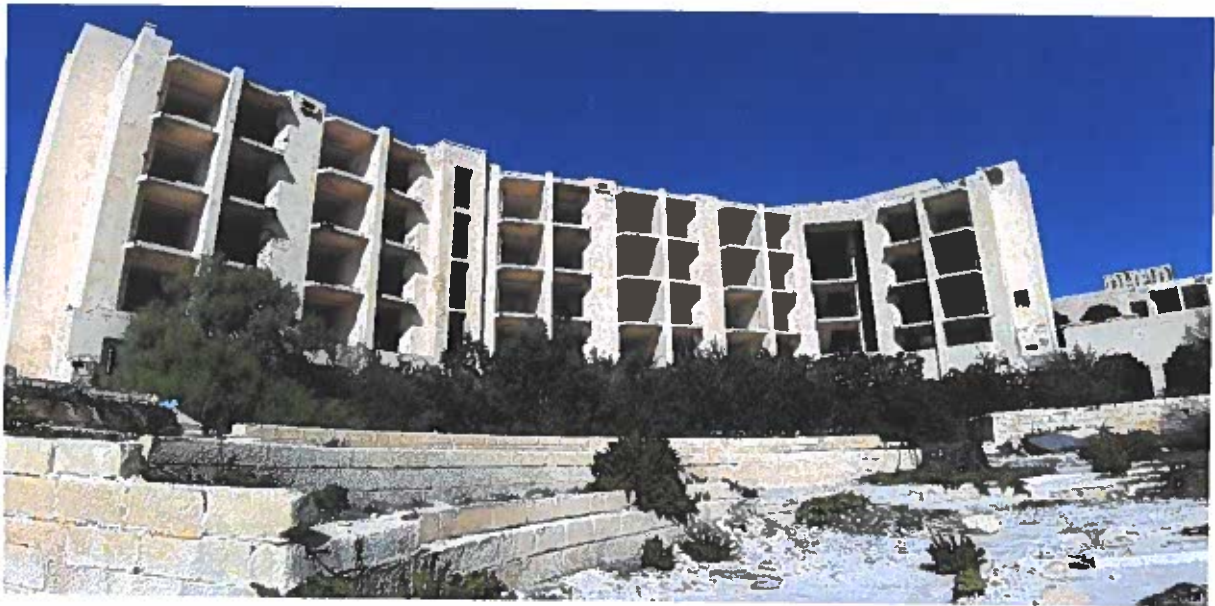
Figure 13 A view of the hotel in the vicinity of St Thomas Tower (overleaf) and showing Zonqor point in the background (top), with the hotel from within the site in its dilapidated state (bottom)
