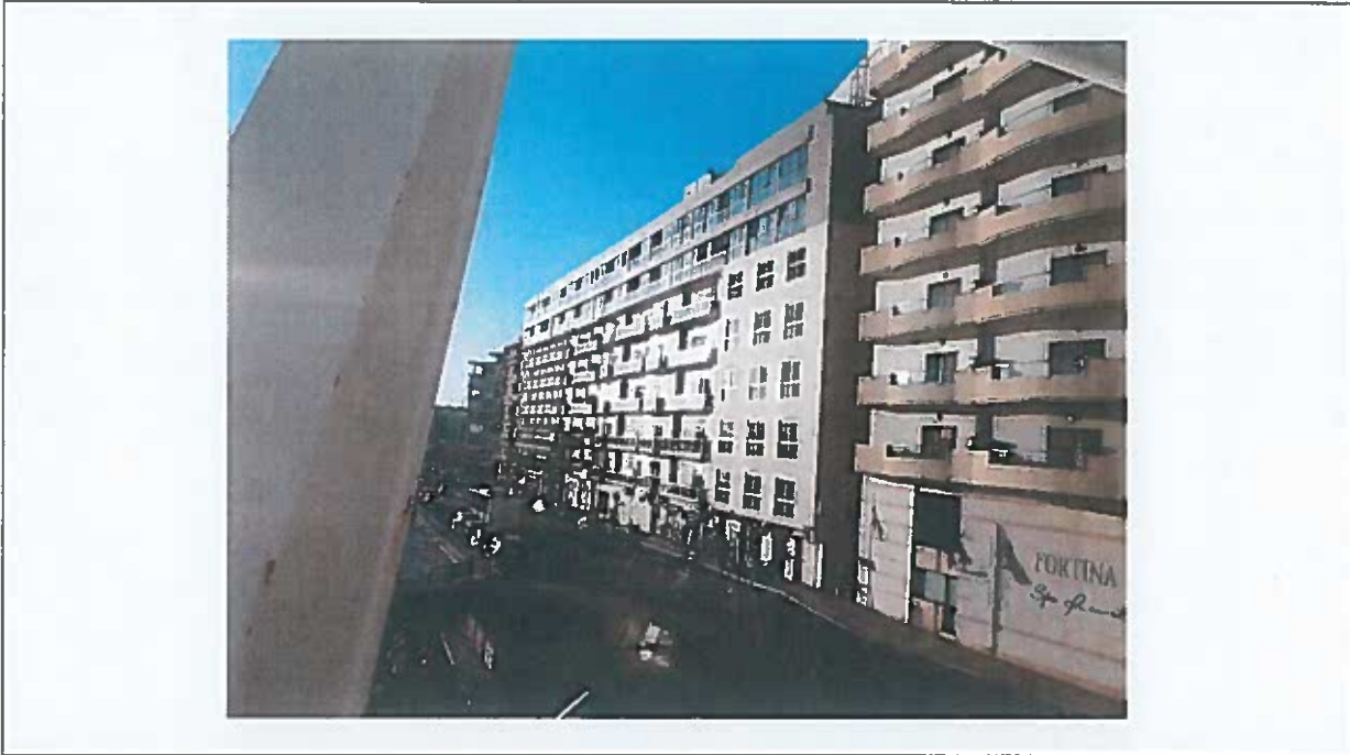
Photo 1: Note existing seafront façade – 8 stories high, note an existing additional floor as recessed from façade.
