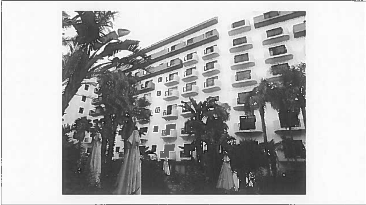
Photo 7: back 8 storey façade of the rear rooms – note pool deck situated at 1 st floor of pool complex.
